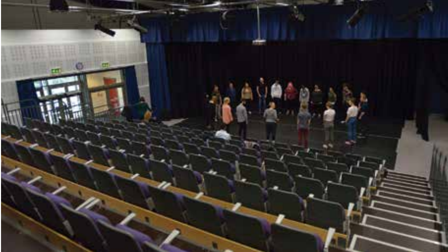
CDEC installed new projection equipment and control systems at Bolton University
