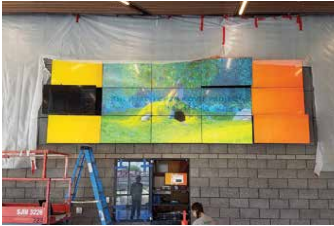
A tvONE CORIOmaster video wall being installed in a technical school
